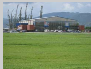
Trincity Business Park
